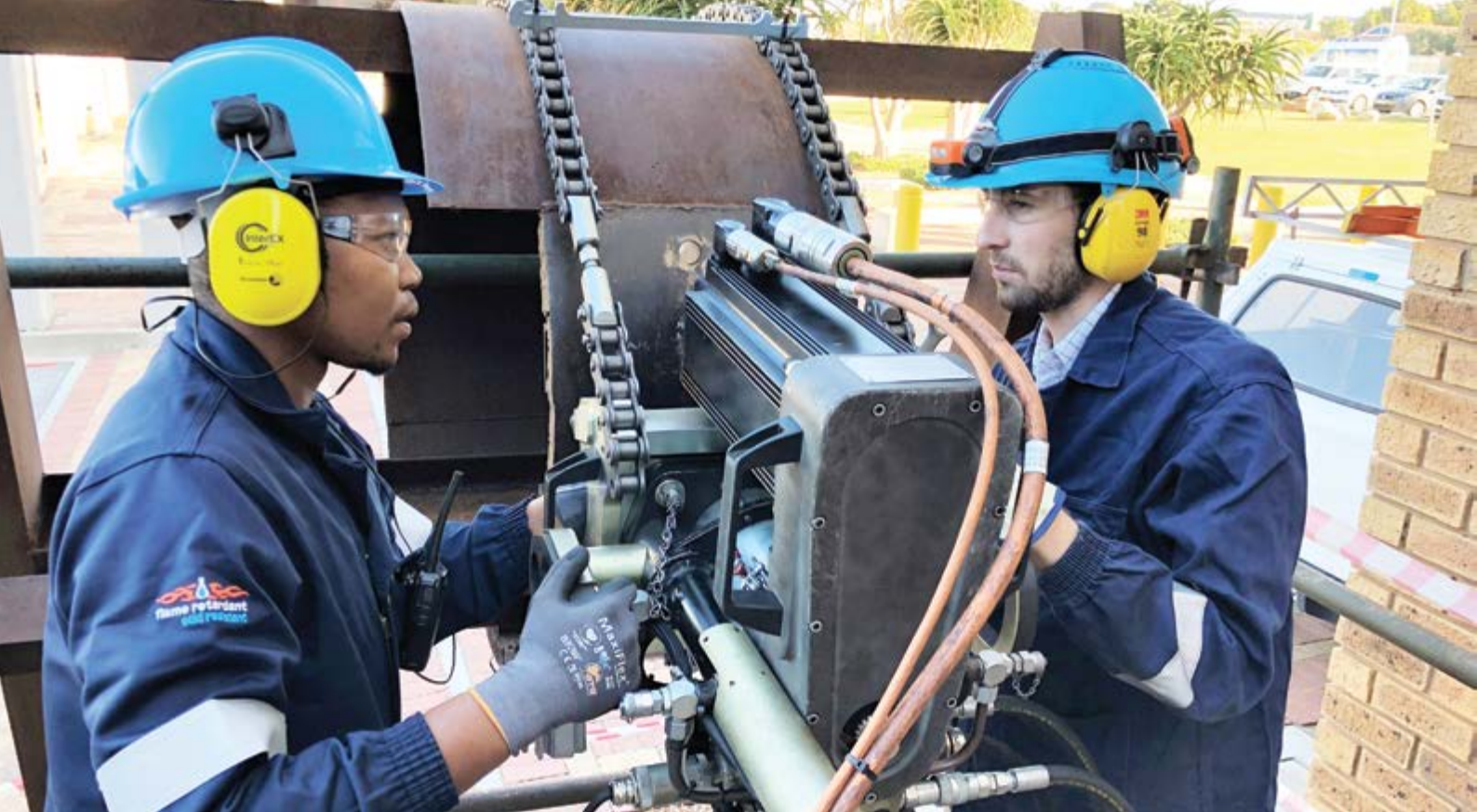
eNtsa engineers prepare for site application with Weldcore® technology
