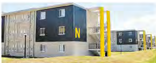
GEARING UP: All new Nelson Mandela University residences are designed with sustainability as a priority. Picture: SUPPLIED
