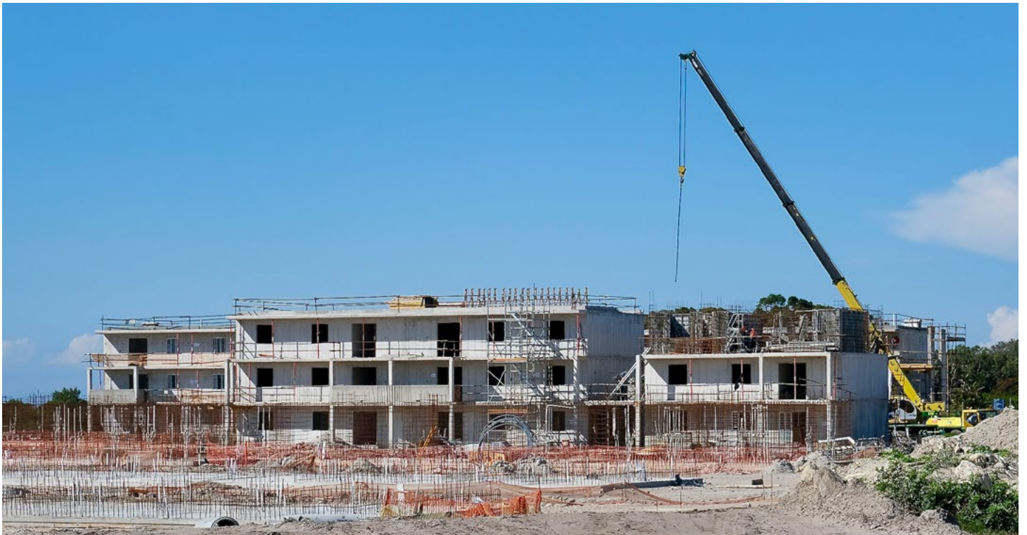
Work on a new 1000 bed residence should be complete later in 2022
