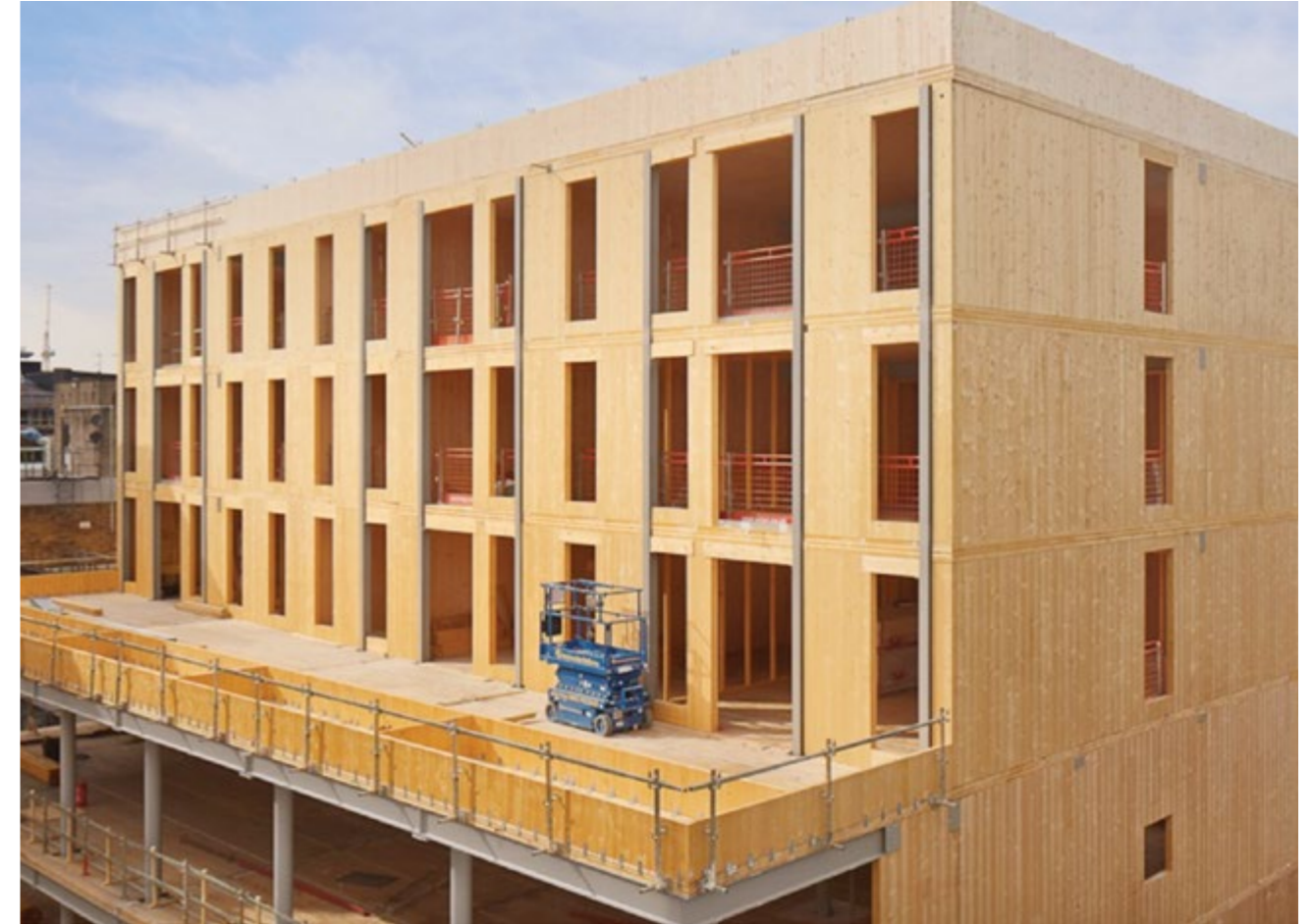
Curtain Place, by Waugh Thistleton Architects, is a six-storey CLT development situated in the heart of Shoreditch, London. Photo: Waugh Thistleton Architects
