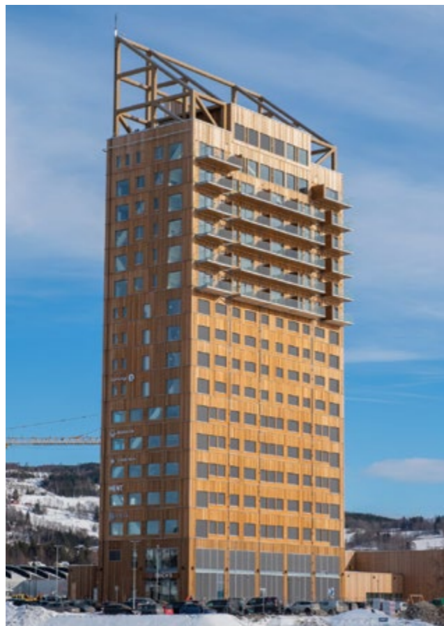
Mjøstårnet – Moelvern Wood Construction. The 85.4m high building was opened in March 2019 and is officially the world’s tallest timber building. Mjøstårnet has a combined floor area of around 11 300 square metres. The building has 18 storeys that include apartments, a hotel, offices, a restaurant, a rooftop terrace and common areas. Photo: Moelvern Wood Construction
