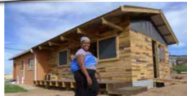
Spaza shop from recycled pallets for owner Thembakazi Thelma (pictured here), Joe Slovo community
