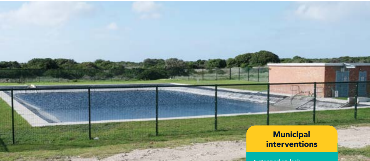
Return effluent retention pond and pump station
