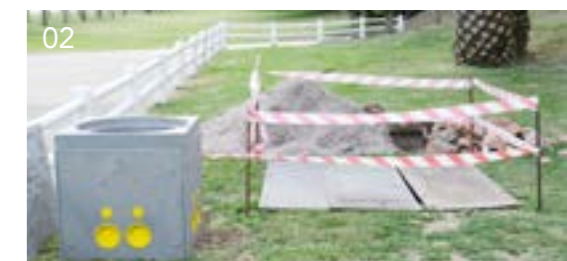
01 New return effluent irrigation system installed on a rugby field 02 Water meter installation with new composite drop-in valve or meter chamber
